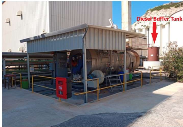
Auxiliary Boiler and Diesel Buffer tank
